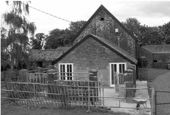
Office before and after
