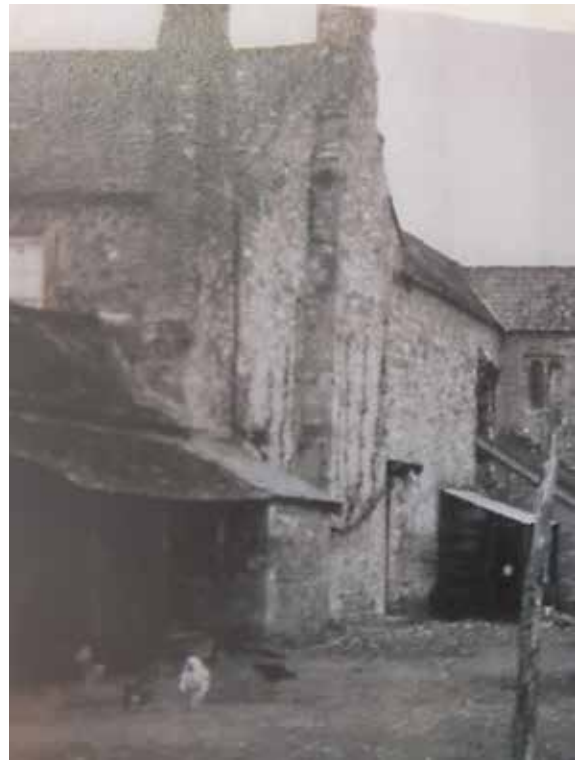
Dangerous chimney stack
